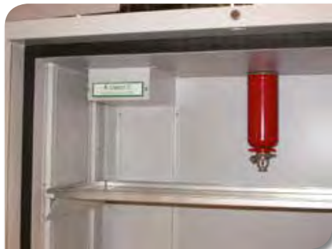
Fire-extinguisher installed in a safety cabinet
