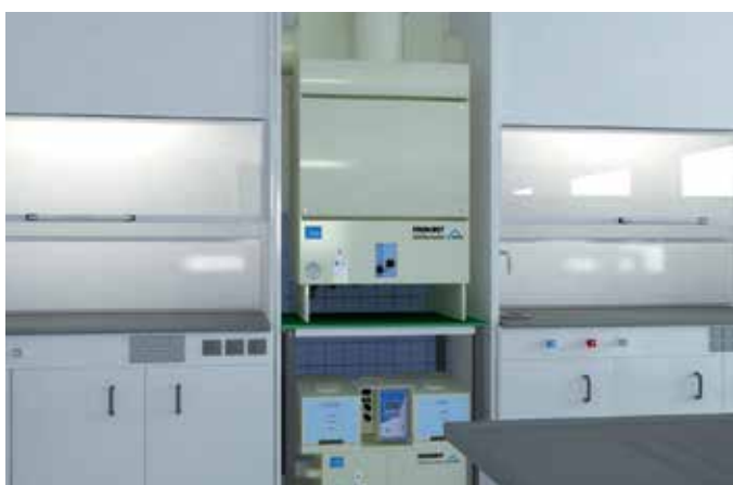
Figure 3 Fume cupboards with FRIDURIT fume scrubber and neutralisation unit
